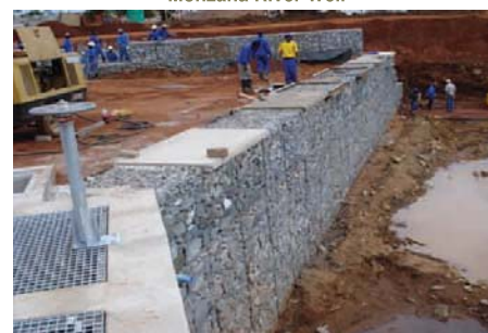
Re-enforcement of base and Gabion Protection - Monzana River Weir
