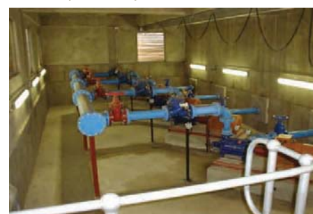
Completed Pump Station at Monzana River
